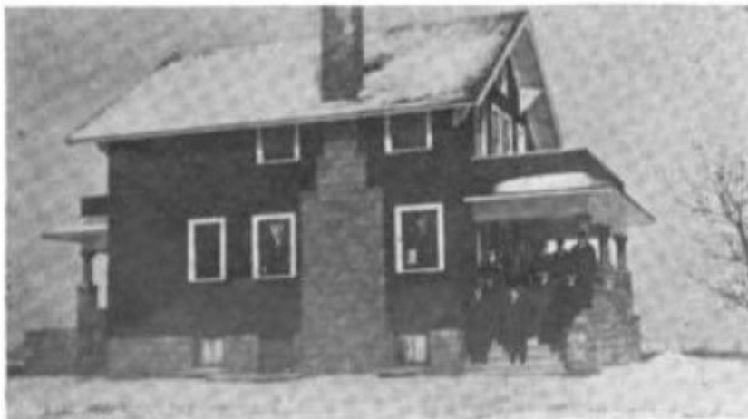
W. G. Alexander was the first Commodore elected in our current clubhouse, November 1911. This photograph depicts the building in February 1914 in Rudder Magazine . The leadership is posing on the east porch.
